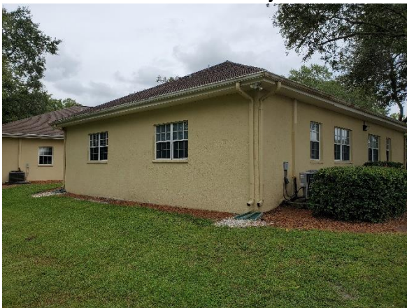
Exterior View of Subject
