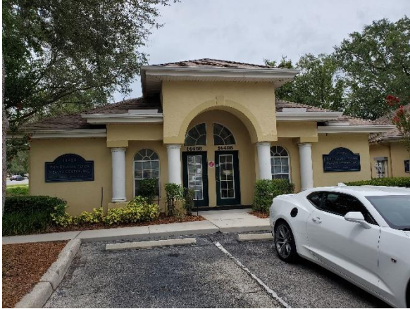
Exterior View of Subject
