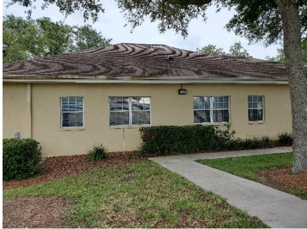
Exterior View of Subject
