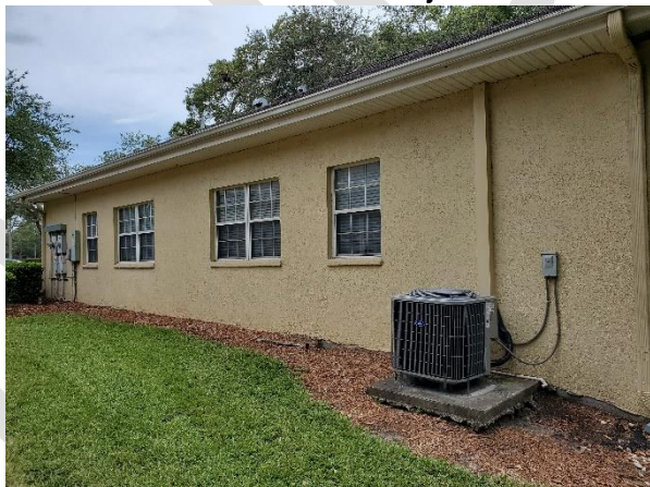
Exterior View of Subject
